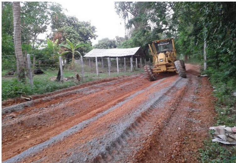
SOIL STABILIZATION OF THE UPPER GROUND LAYER OF THE LOCAL ROAD BY THE "PARAGON" TECHNOLOGY
